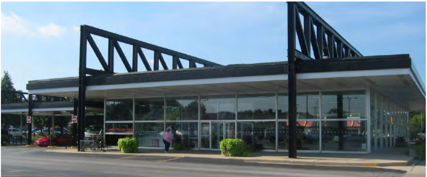
Villa Park Bank Today
